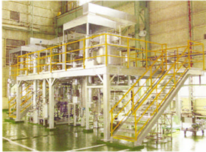
Figure 1. Pilot plant for methanol production from biomass.
