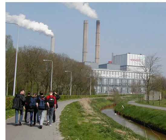
Amer power plant of Essent 1245 MW e (net) and 600 MW th pulverised coal fired 2 CHP units AMER-8 and AMER-9
