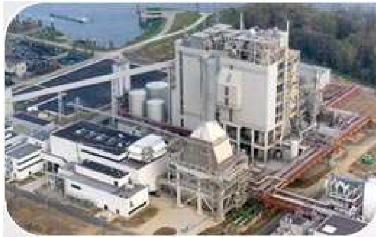
NUON Buggenum coal/biomass fired plant (NL): 250 MW e
