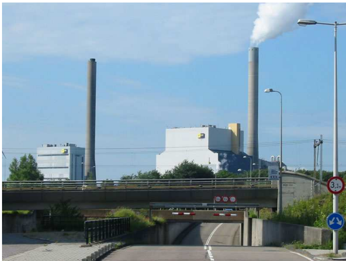
Hemweg power plant of NUON 630 MW e (net) pulverised coal fired
